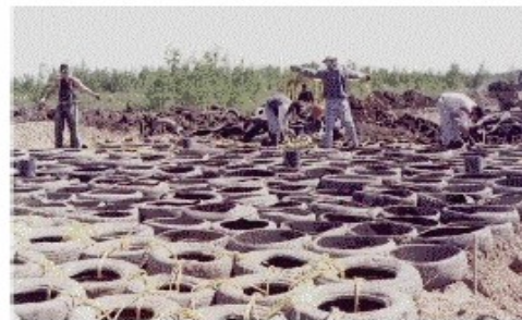
Earth Retaining Wall Using Scrap Tires
